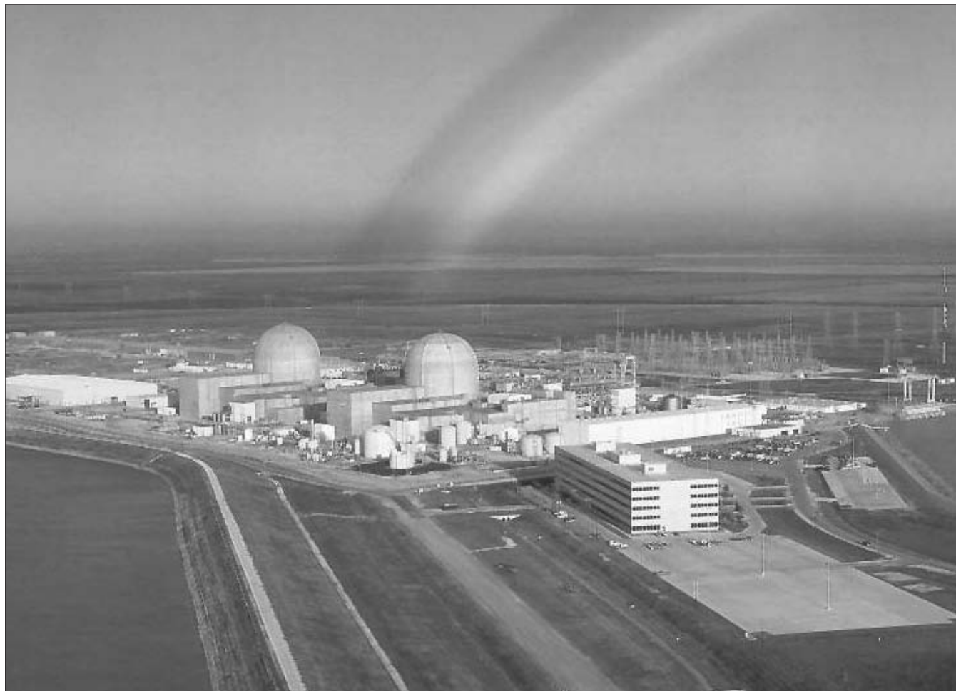
Photo Courtesy South Texas Nuclear Power Plant
